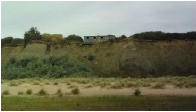
Comments on cliff top structure: None
