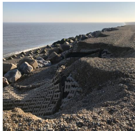
Figure 9: Interlocking block revetment failure, sub-unit A in January 2019 (Provided by G Watson, Environment Agency).
