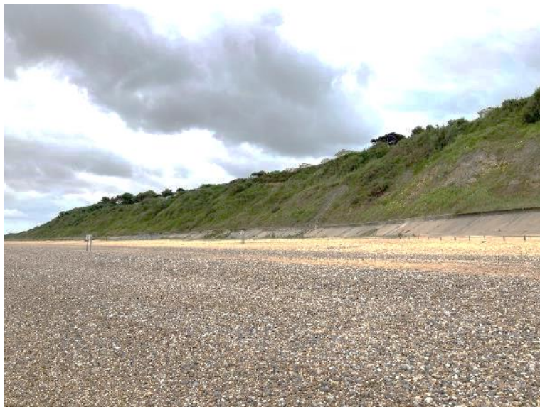
Figure 3.1n. CBU 8. Azure Sea north. The cliff is degraded and well-vegetated with a mantle of debris apron that is marginally stable. Periodic activity comprises slumping of debris apron over the toe protection measures in response to wet weather. Seepage is often observed draining over the concrete apron along this section of coast. Note the particularly wide beach at this southern extent of Corton, which monitoring shows has accreted in the last 5 years.
