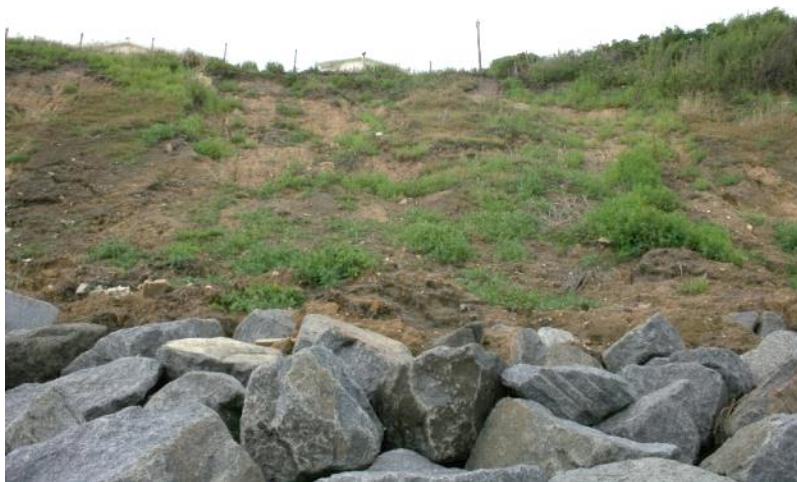
Figure 3.1f. CBU 3. Degraded cliff fronting the Wy-Wurry Caravan Park. This section of cliff experience headscarp retreat and slumping of debris in the storm surge of 3rd April 2021. The Cromer Till is below the level of the rock armour, with the cliff formed of Corton Sand with a thin cap (<1 m) of Lowestoft Till.
