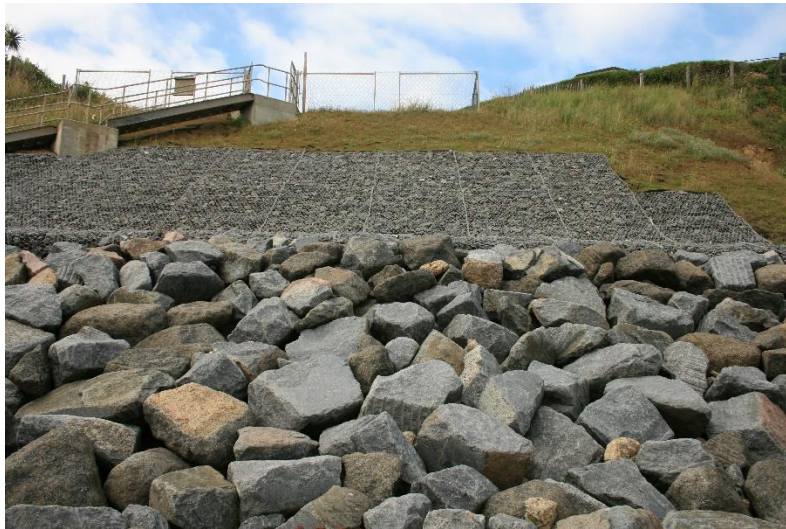
Figure 3.1e. CBU 2. Defended cliffs at Baker's Score. This section of cliff has rock armour below and above a concrete walkway. The cliff has been regraded and protected with gabion baskets.
