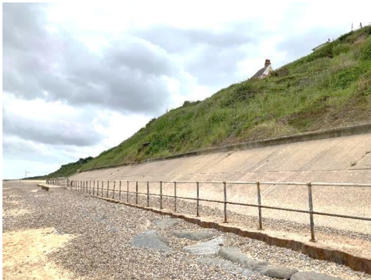
Figure 3.1m. CBU 7. Cliff House to Azure Sea. The cliff is degraded and well-vegetated with a mantle of debris apron. Periodic activity comprises slumping of debris apron in response to wet weather.
