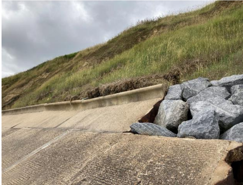
Figure 3.1h. CBU 4. Degraded, locally active cliff fronting the northern part of the Tingdene caravan site. The cliff is formed of Corton Sand with a thin cap ( <1 m) of Lowestoft Till. Recent activity comprises slumps over the concrete apron and toe protection. Note damaged sections of concrete apron have been infilled with rock. Sheet piles have been used at the edges of the concrete slabs to stop water washing beneath.
