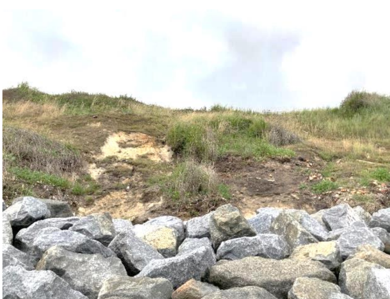
Figure 3.1g. CBU 4. Degraded, locally active cliff fronting the northern part of the Tingdene caravan site. The Cromer Till is below the level of the rock armour and the cliff is formed of Corton Sand with a thin cap (<1 m) of Lowestoft Till and made ground. Note the bricks in the debris that mantles the cliff. Recent activity comprises small slumps of this debris on the lower cliff. The upper cliff is well-vegetated and degraded.
