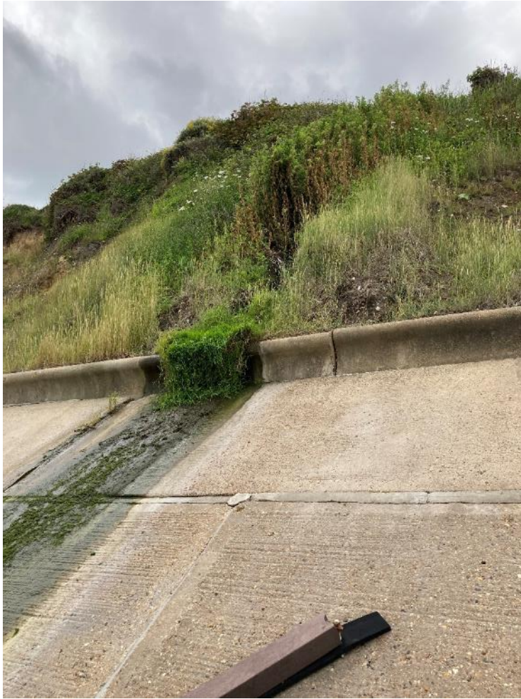
Figure 3.1j. CBU 5. Seepage from drainage outfall from upper cliff at the northern part of the Warner holiday camp, south of Tibbenham's Score. The cliff is degraded and well-vegetated. It is mantled with debris that is saturated with water and which has pushed out the wave return wall. A car park is present on the cliff top, which is not covered by the deep drainage scheme.
