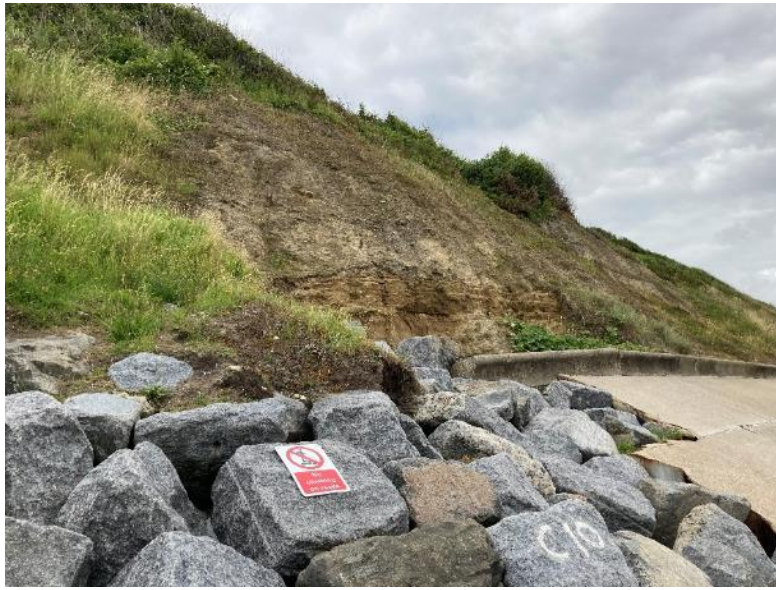
Figure 3.1l. CBU 6. Warner holiday camp south. The cliff is locally active, showing areas that are degraded and well-vegetated, and others that show evidence for recent slumping of debris over the upper rock, and erosion from overtopping waves. The sediments exposed in the base of the cliff comprise around 1 m of banded and gravelly Cromer Till overlain by Corton Sand and a thin cap of Lowestoft Till and Plateau Gravel.
