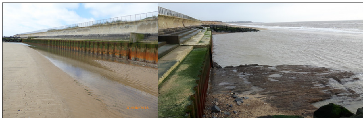
Figure 14 EA Easton Marshes seawall, Left – looking from R8 towards R7 (taken 20 June 2018), Right – lowered level with indications of exposed clay (taken 2 May 2018)
