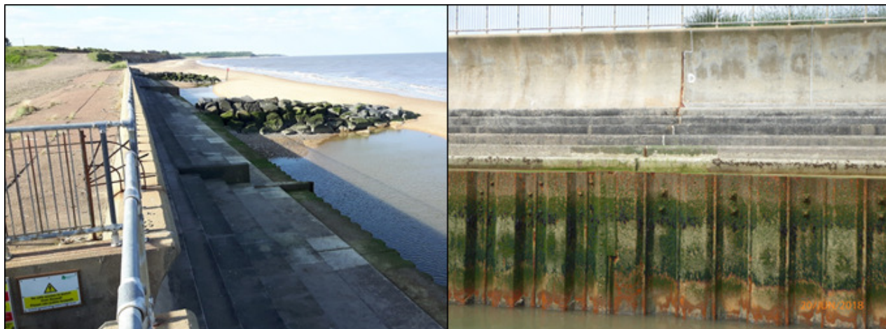
Figure 7 Left - EA Easton Marshes concrete stepped seawall (taken 14 June 2018), Right - where the 1980s seawall extension joined existing seawall (taken 20 June 2018)
