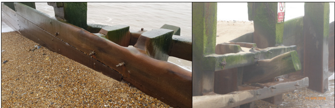
Figure 19 Left & Right - Pictures of wear on groyne T8 (taken 11 April 2018)
