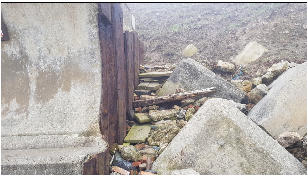
Figure 34 Condition of sheet pile at termination of Easton Marshes seawall and ad-hoc beach access (picture taken 12 April 2018)
