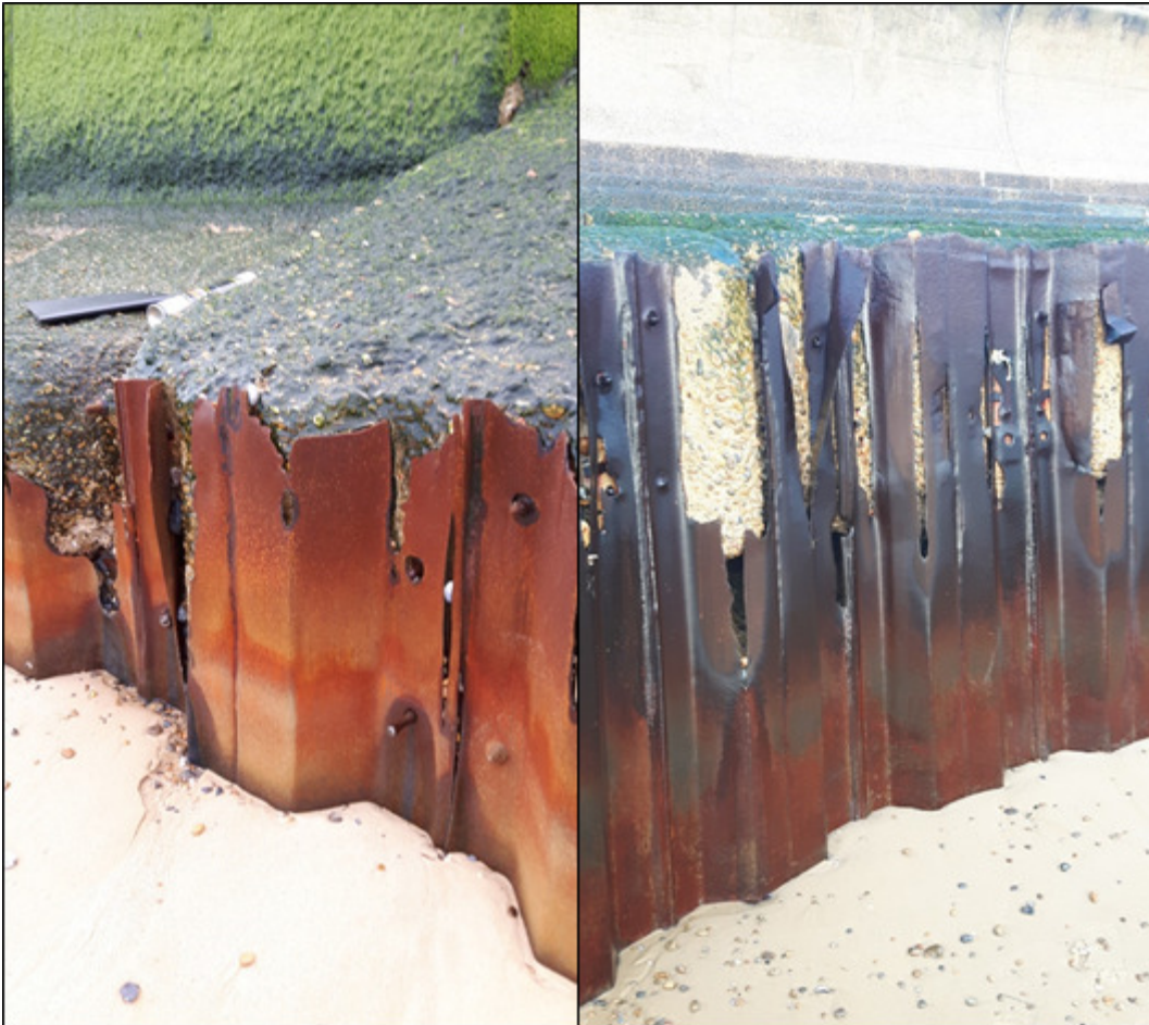
Figure 16 Sheet pile deterioration close to access ramp (Left, taken 16 April 2018, Right, taken 6 March 2018)
