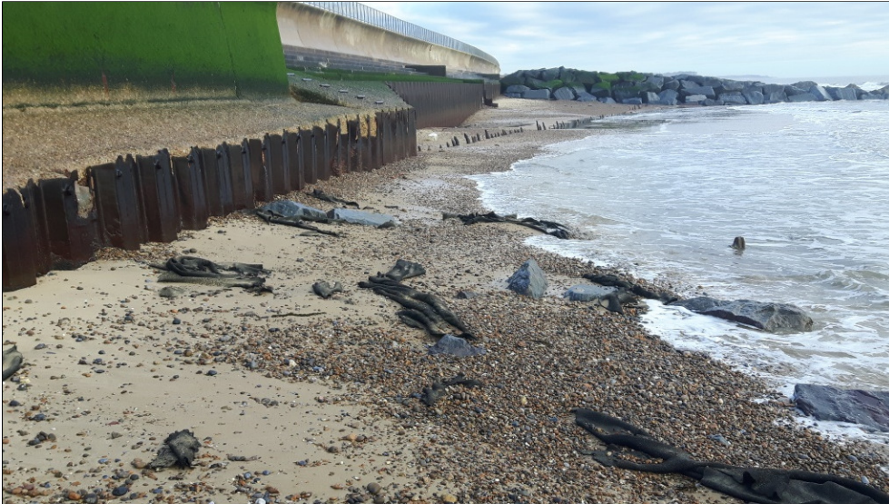
Figure 27 View towards ramp from WDC frontage, geotextile in foreground from previous revetment works, change of section noticeable (picture taken 6 March 2018)
