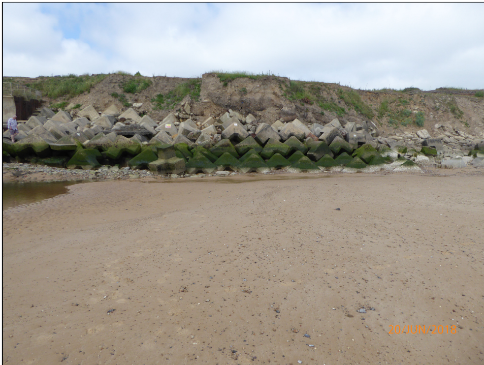
Figure 32 Extent of Tripod armour units (picture taken 20 June 2018)
