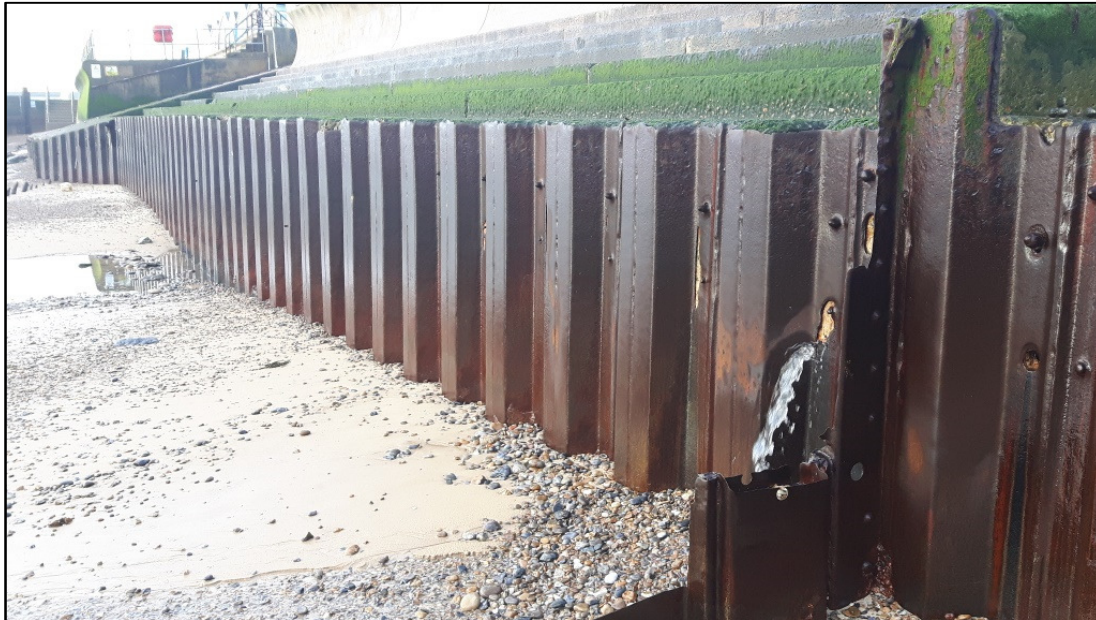
Figure 17 Sheet pile damage close to groyne R5 (taken 6 March 2018)
