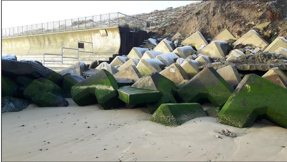
Figure 31 Termination of Easton Marshes seawall protected by Tripod concrete armour units (picture taken 12 December 2017)
