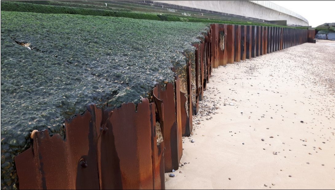
Figure 15 Sheet pile deterioration along EA seawall at location near to access ramp (picture taken 16 April 2018)
