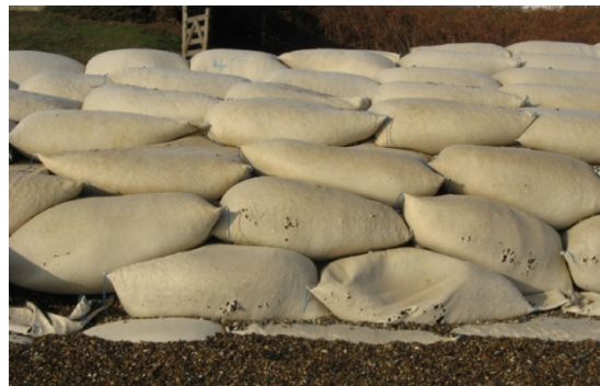
Figure 1.1: The seaward edge of the Phase 1 Geobag layers showing holing from abrasion.
