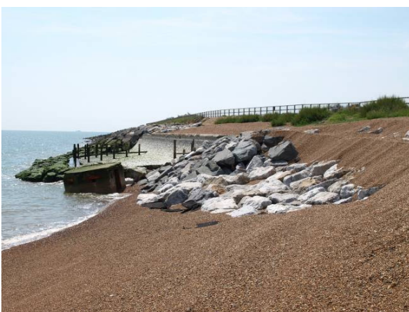
Coastal defences north of East Lane. The wall and apron were observed in the 1992 aerial photos. Note rock armour in foreground to limit outflanking. Aerial photos show this material is occasionally covered by gravel.
