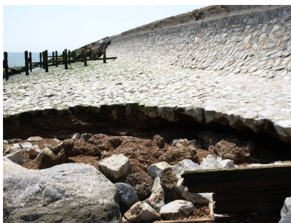
Undercutting of the apron has occurred behind the pill box.
