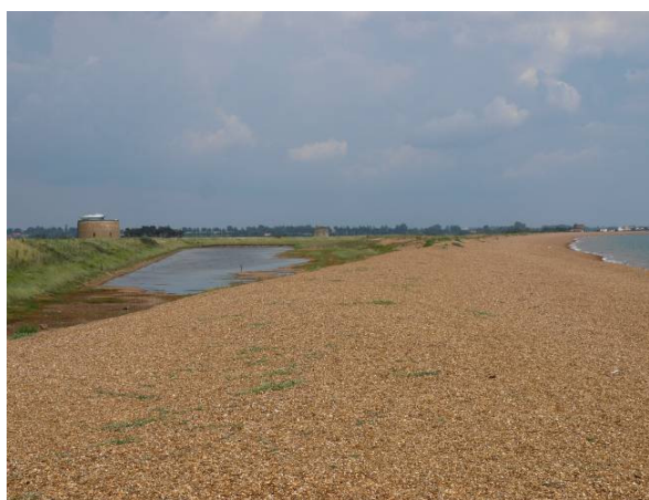
Hollesley Bay, healthy beach looking north. Note saline lagoon formed between beach ridges and coastal flood embankment. The different alignment of the beach and the embankment suggest significant beach progradation.
