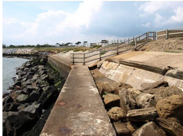
Defences on the south side of the East Lane headland. Note rock armour covering toe of revetment apron
