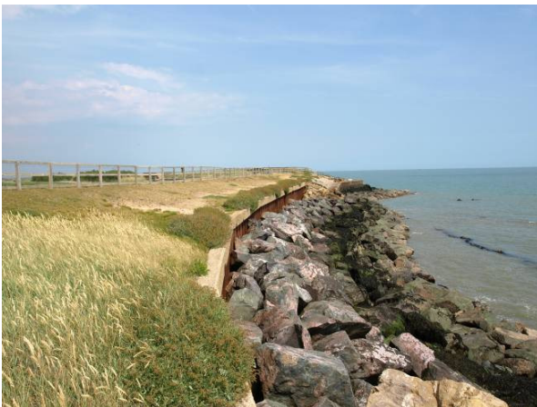
Sheet piles installed in 2009 following overtopping of rock armour and cliff recession.
