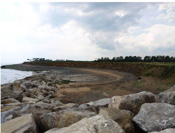
Rock armour end structure, bay formed behind the armour and thin and narrow beach. Tide line shows deeply-indented London Clay shore platform.
