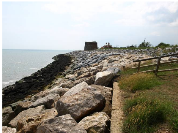
Continuous rock armour to Martello tower.
