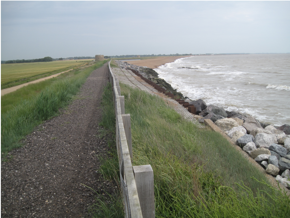
Fig.11A: Looking northwards towards SSB. Serial coastal protection (rock armouring) along the old Flood Bank.
