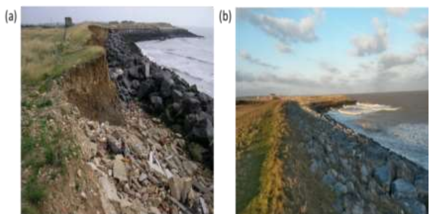
Figure 3.6: South of East Lane point (a) before repairs in 2005; (b) after repairs in 2015 (from approximately the same vantage point).
