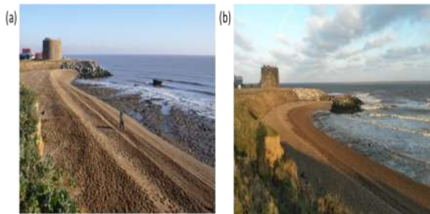
Figure 3.11: Beach conditions south of the rock armour fishtail groyne termination in February: (a) 2007; and (b) 2015.
