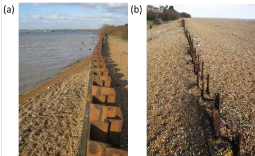
Figure 4.10: Sheet pile defences at the mouth of the Deben Estuary: (a) good condition; and (b) badly corroded.
