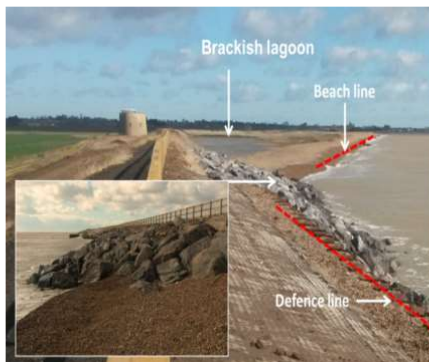
Figure 3.18: Completed defences in March 2015. The inset shows the defence termination with the natural shingle beach.
