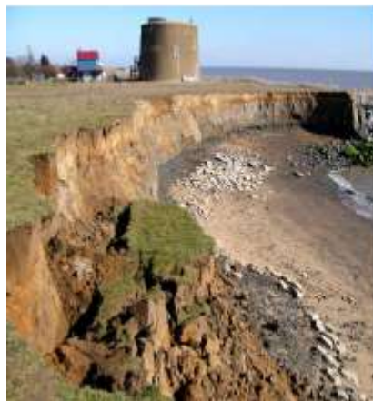
Figure 3.9: Erosion at the southern termination of the defended frontage in 2006.
