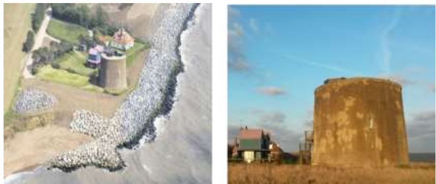
Figure 3.1: Martello Tower at East Lane, Bawdsey (with Phase 2 defences in place).
