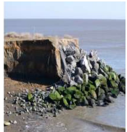
Figure 3.9: Erosion at the southern termination of the defended frontage in 2006.
