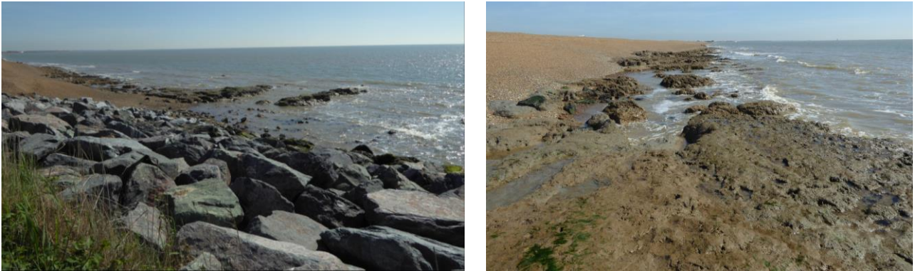
Figure 5 Exposure of underlying London Clay at northern end of East Lane defences. Taken June 2017.
