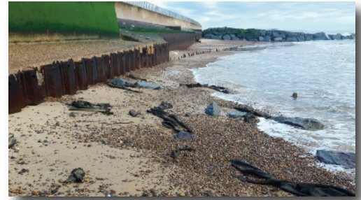
Photo showing defence deterioration at Southwold, 2018
