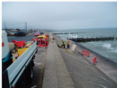
Repairs to the lifted slabs at Bacton and Walcott
