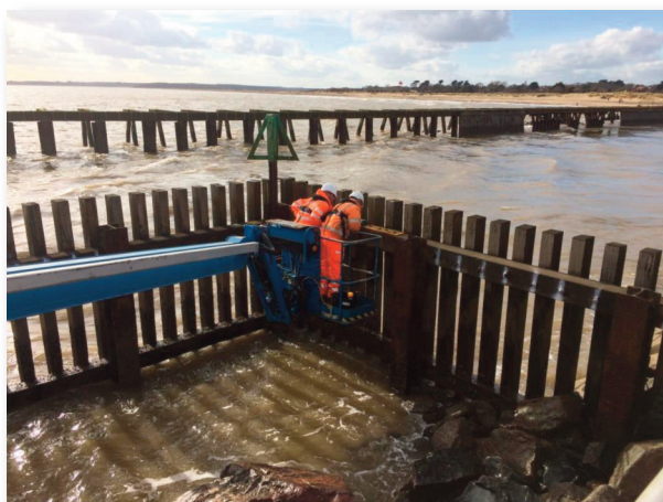
The Water Management Alliance inspecting and repairing Southwold fender
